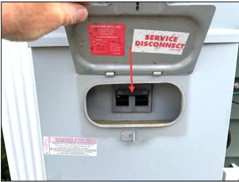
Main electrical shut off switch.
