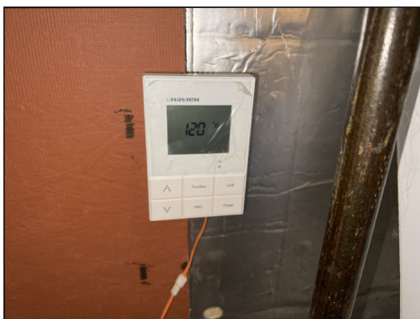
Water heater thermostat currently set at 120F. Between 110F - 130F is the industry standard.
