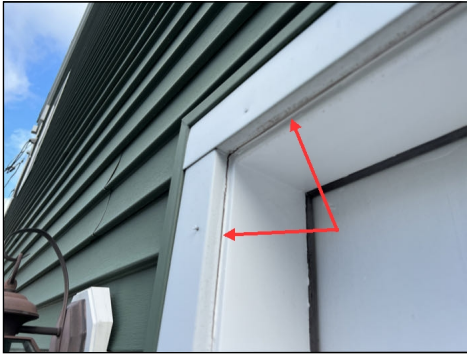
Deteriorated and split caulking observed, maintenance is advised where necessary.
