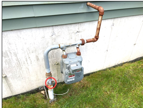
Main gas shut off valve.
