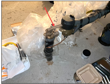
Main water shut off valve.
