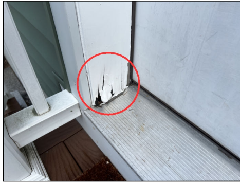
Areas of wood decay were observed on the door trim at the side entrance and the entrance door. Replacement of all decaying areas where necessary is advised from a qualified contractor.
